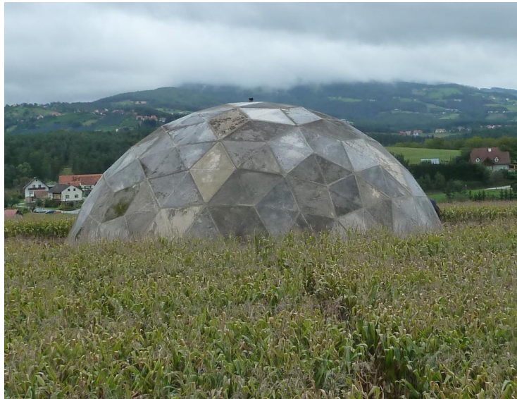
Figure 7: sounddome as hemisphere, 20 m diameter in cornfield
